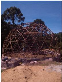
The presentation dome is the first one to be constructed and is shown here at its first stages of foundations and timber dome frame.
